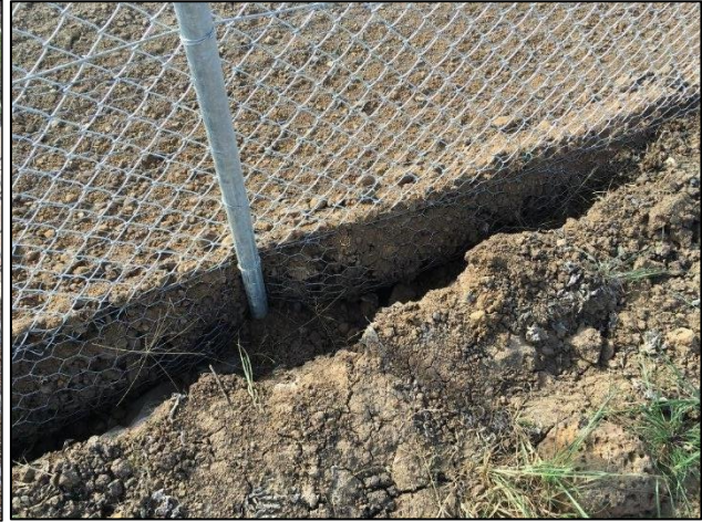
Plate 12. Rabbit proof fence constructed surrounding the offset site (Ecology and Heritage Partners 03/08/2020).
