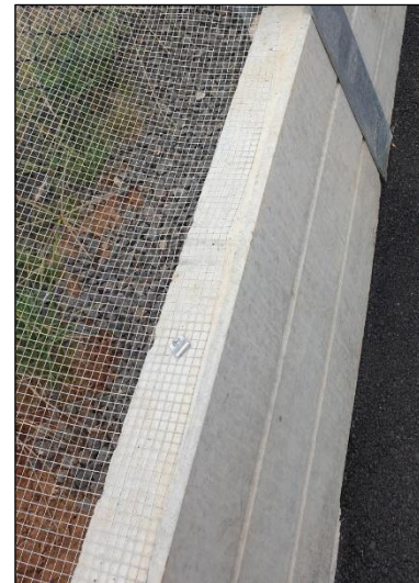
Plate A5.4. Rabbit proof mesh attached to the cyclone fence and secured to retaining wall (Photo provided by Citius 8/04/2022).
