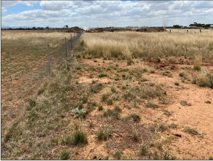
Plate B4.1. Rabbit proof fence along the north-west boundary (Ecology and Heritage Partners Pty Ltd 10/02/2022).
