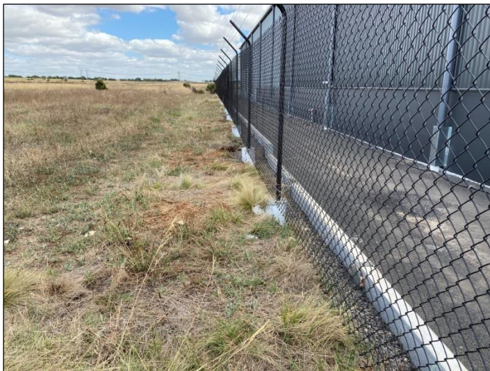
Plate C4.1. Cyclone fencing with gap at the base (Ecology and Heritage Partners Pty Ltd 10/02/2022).
