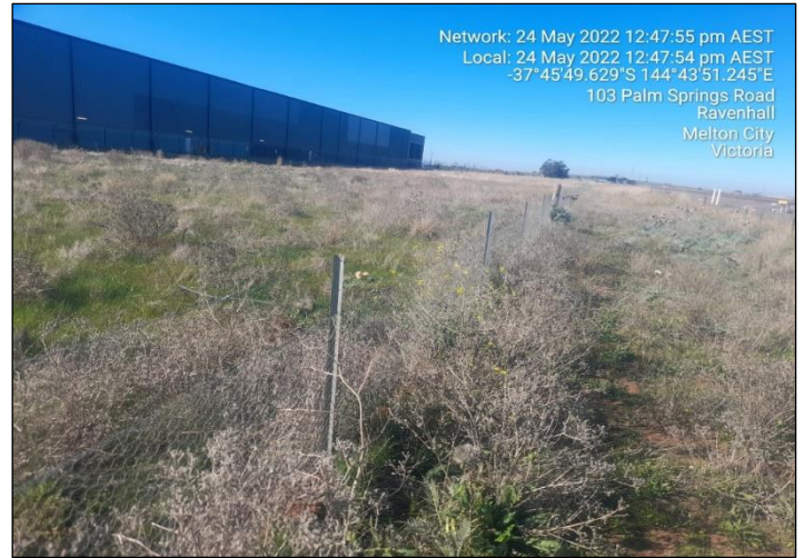
Plate A5.6. Repaired broken wire in zone 2D (Photo provided by Citius 25/05/2022).
