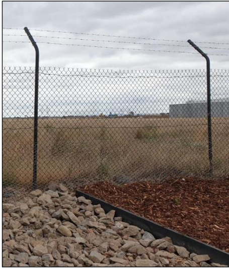
Plate A5.1. Rabbit proof fencing buried and attached to the cyclone fence (Photo provided by Citius 8/04/2022).
