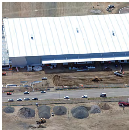
Quarry Industrial Estate, 2 Bellevue Circuit, Greystanes
