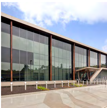
Quarry Industrial Estate, 6 Bellevue Circuit, Greystanes
