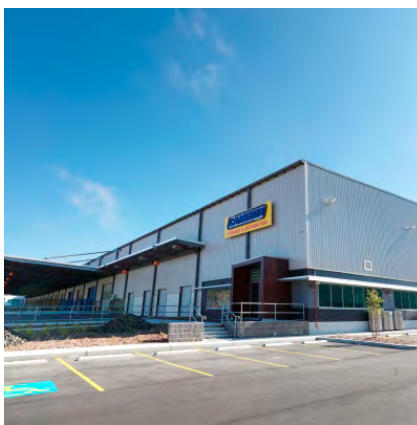
Quarry Industrial Estate, 2-6 Basalt Road, Greystanes
