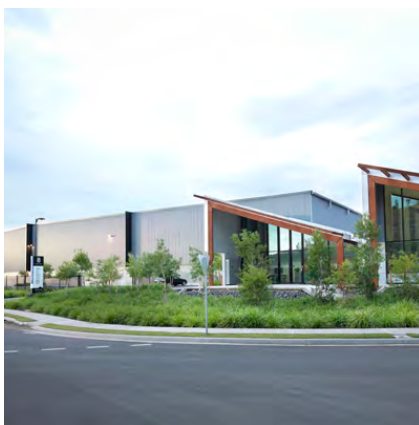
Quarry Industrial Estate, 8 Basalt Road, Greystanes
