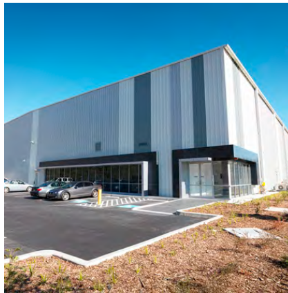
Quarry Industrial Estate, 5 Basalt Road, Greystanes
